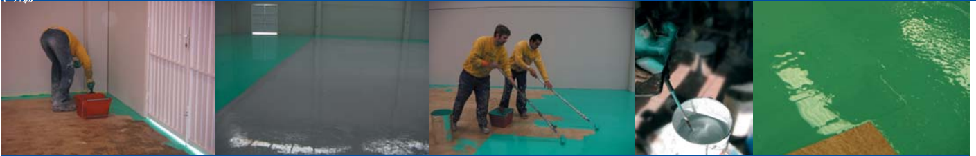
Industrial floor treatment and coating using COLODUR aliphatic Polyurethane single component resin.
